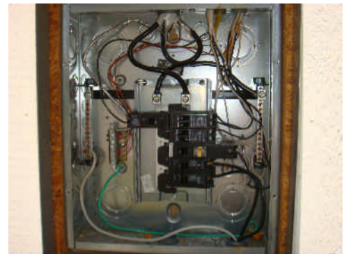
Arc-fault circuit interrupter breaker.
