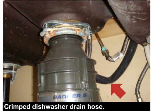
Crimped dishwasher drain hose.
