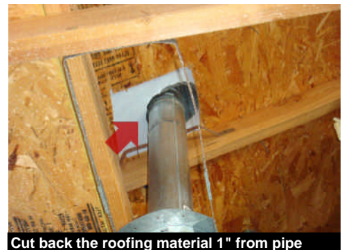
Cut back the roofing material 1" from pipe
