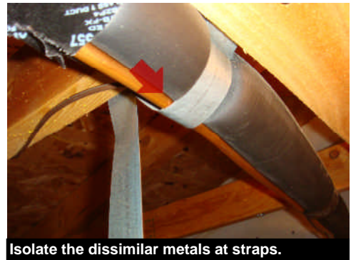
Isolate the dissimilar metals at straps.
