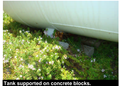
Tank supported on concrete blocks.
