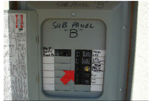
Arc-fault circuit interrupter breaker.
