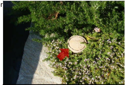
Suspected pool fill valve.
